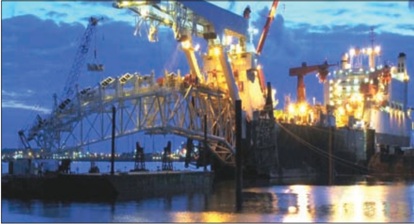
The Solitaire in Rotterdam harbour can lay pipes for oil and gas and oceans to depths over 2700 m using the S-lay method over its stinger. This floating factory ship with a length of 300 m (excluding stinger) accommodates 420 men. (Photo: DirkJan).
