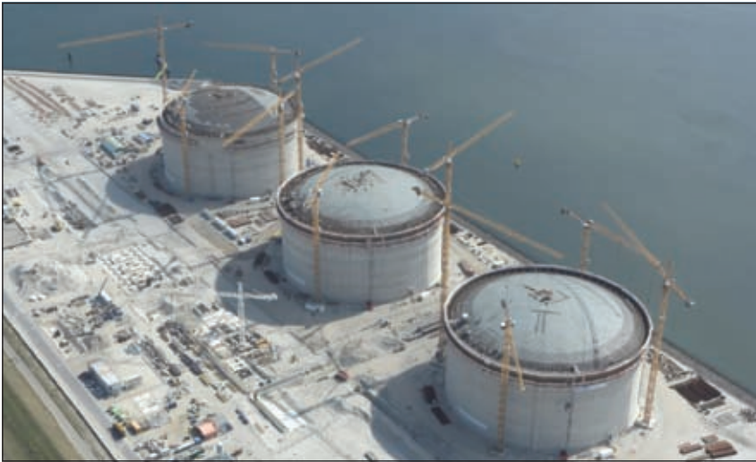
Figure 4a LNG Gate terminal construction in Rotterdam port started in 2009 with three huge storage tanks. They will be ready to land LNG imports from 2012 onward. The LNG terminal will have an initial throughput capacity of 12 bcm per year, which requires about 150 shipments a year (Photo: GATE).
